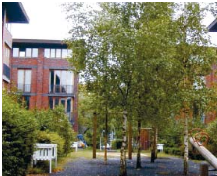
Courtyard development, incorporating landscaping can assist energy efficiency
