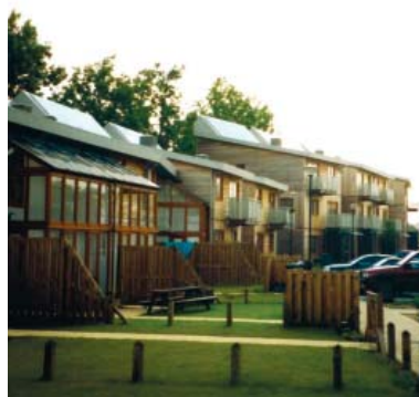
Solar panelling on house roofs in Berkshire
