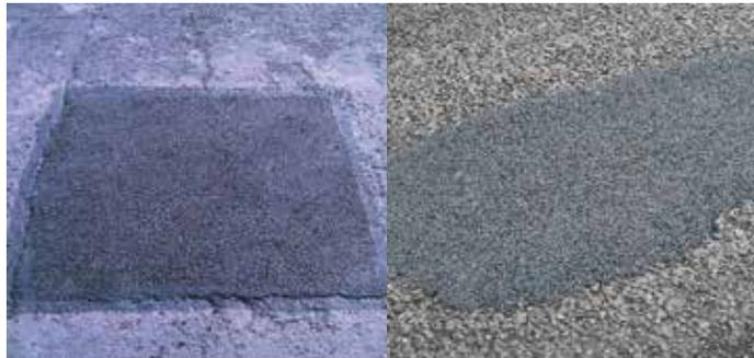
bituminous binder. The hole is then filled with a hot bitumen-bound material which is raked and compacted.
